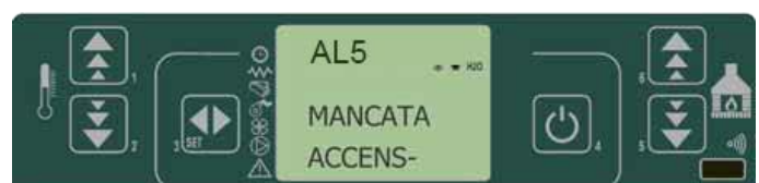
fig. 39 control panel - failed ignition alarm
