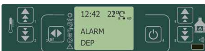
fig. 37 control panel - auger safety pressure switch alarm
