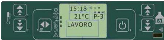
fig. 25 control panel - operating condition
