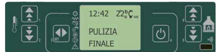
fig. 41 control panel - power failure
