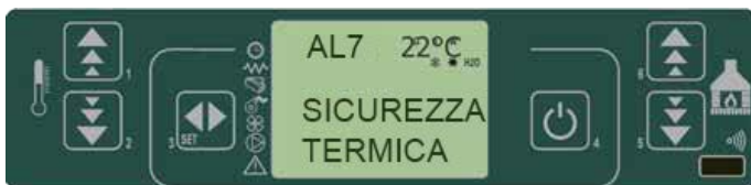
fig. 42 control panel - general thermostat alarm
